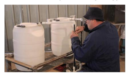
I'm using the PVC tape because it makes the connection with the taps more much easier to do.
