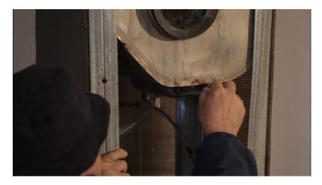
Now I'm introducing the plug-in cable inside the box where I will make the connections between the socket, thermostat and the switch.
