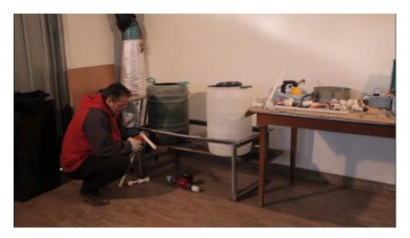
I drill holes at the bottom of the both barrels for the taps, which will connect the barrels.
