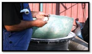
On the margin of the black tube I apply silicone before installing the fiberglass dome in place.
