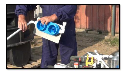
All you need to do the pvc piping are a couple of fittings, a pvc welding tool and a tool to cut the pvc pipe.
