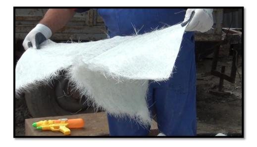
To obtain a strong surface, I need to apply a couple of layers of rosin and fiberglass.
