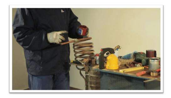
To secure the coil in place, I will use this steel ribbon.
