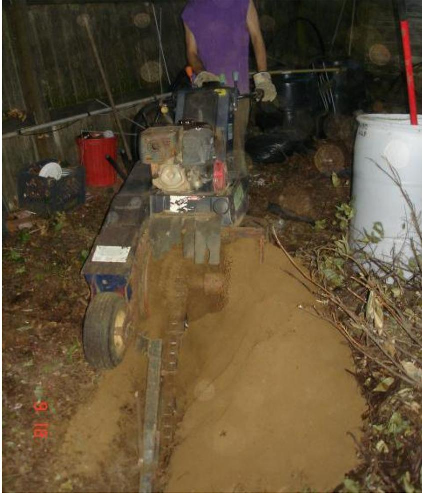
So the trenches went in and great care was used to not damage any of the polyethylene loop pipes.
