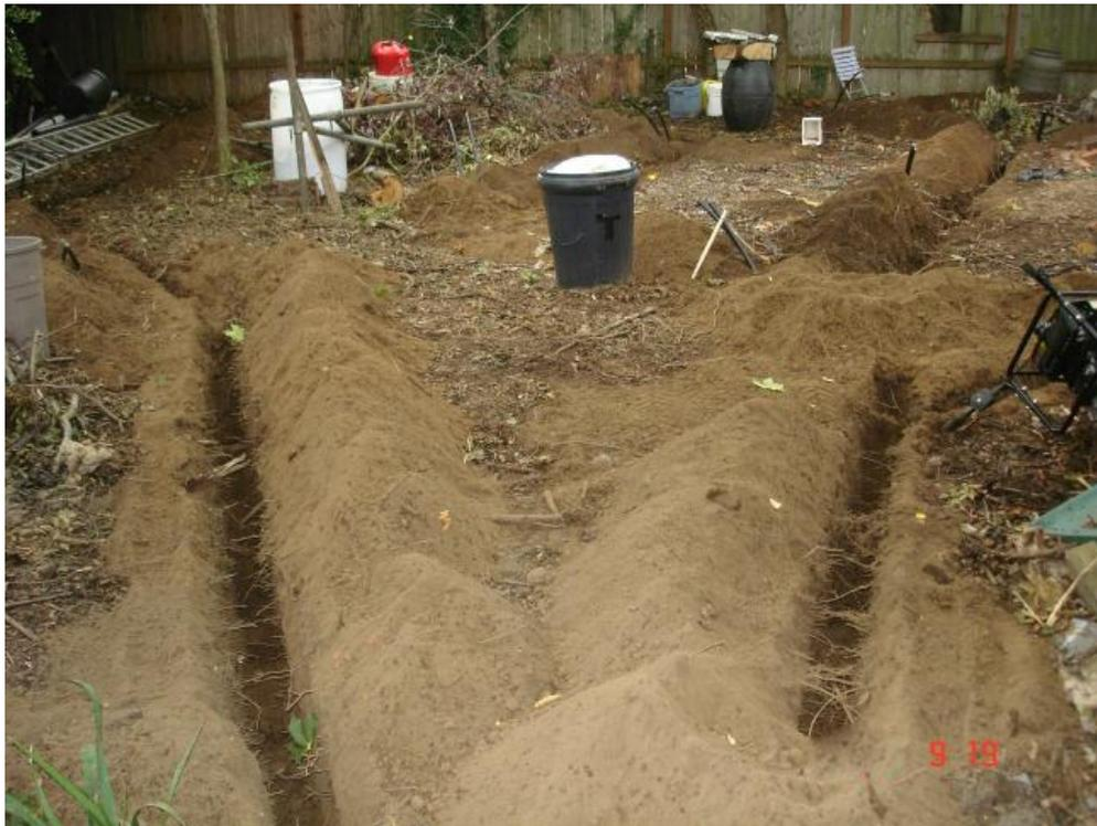
I found that it really pays to run the trencher as close as possible to the plastic pipe, without hitting the plastic. Making corrections for a wide space (I had many) has been very time consuming.
