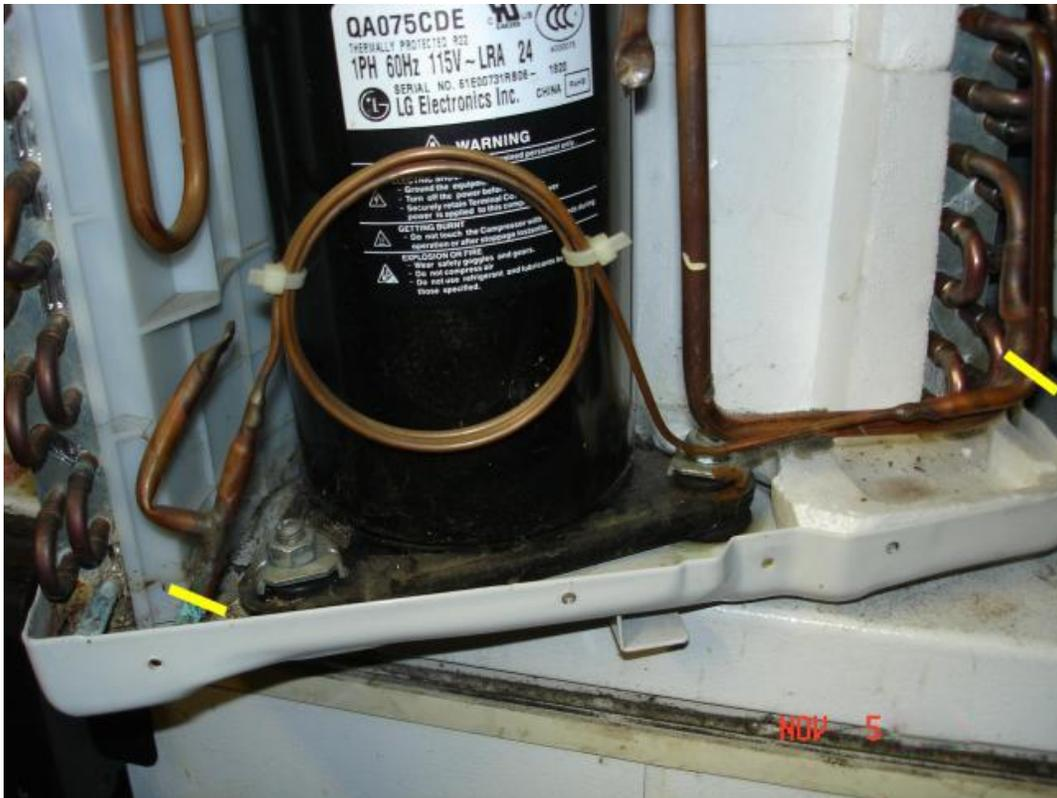
This tiny coil is called the 'cap tube', no relation to the capacitor...
