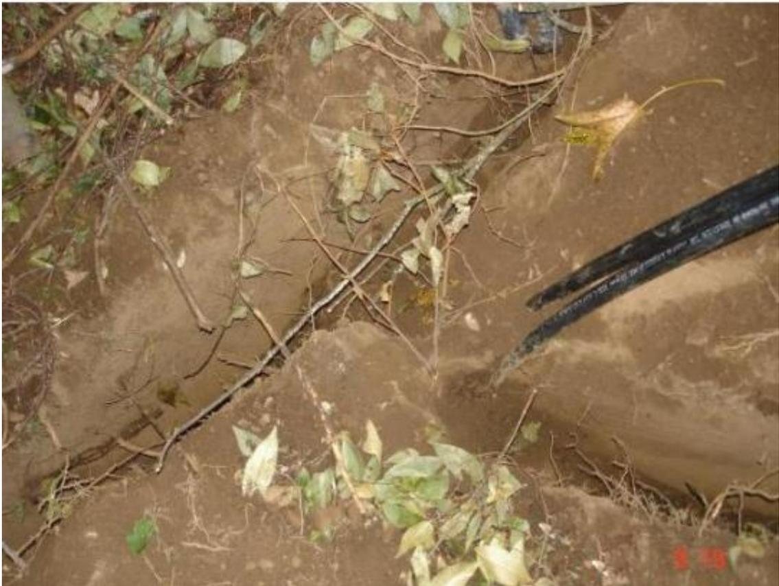
...the pic on the bottom shows digging the trench next to the loop pipe.
