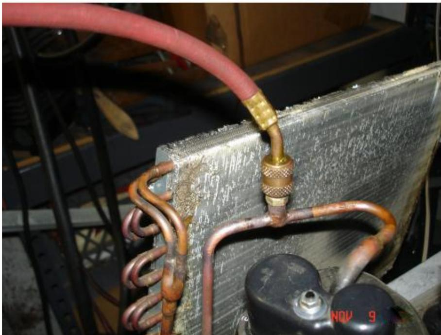
The bottom photo shows the vacuum hose connecting to the previously brazed Schrader valve on the AC unit.
