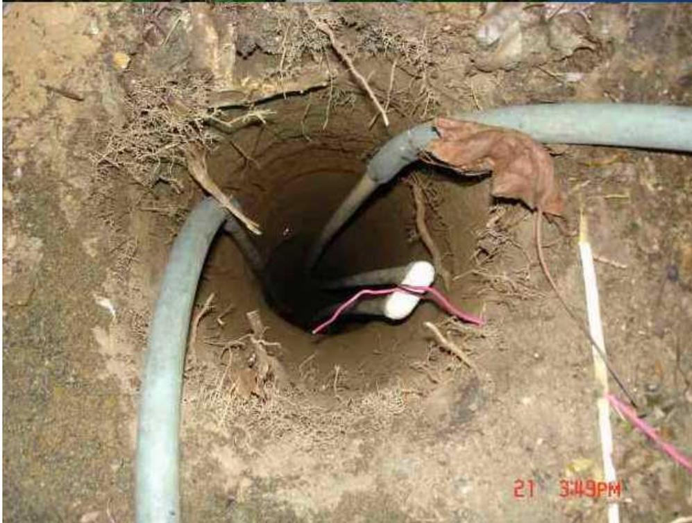
this shows the hole I'm doing the tests in. I used CPCV pipe (not recommended) with a double-loop (not much advantage over a single loop)...
