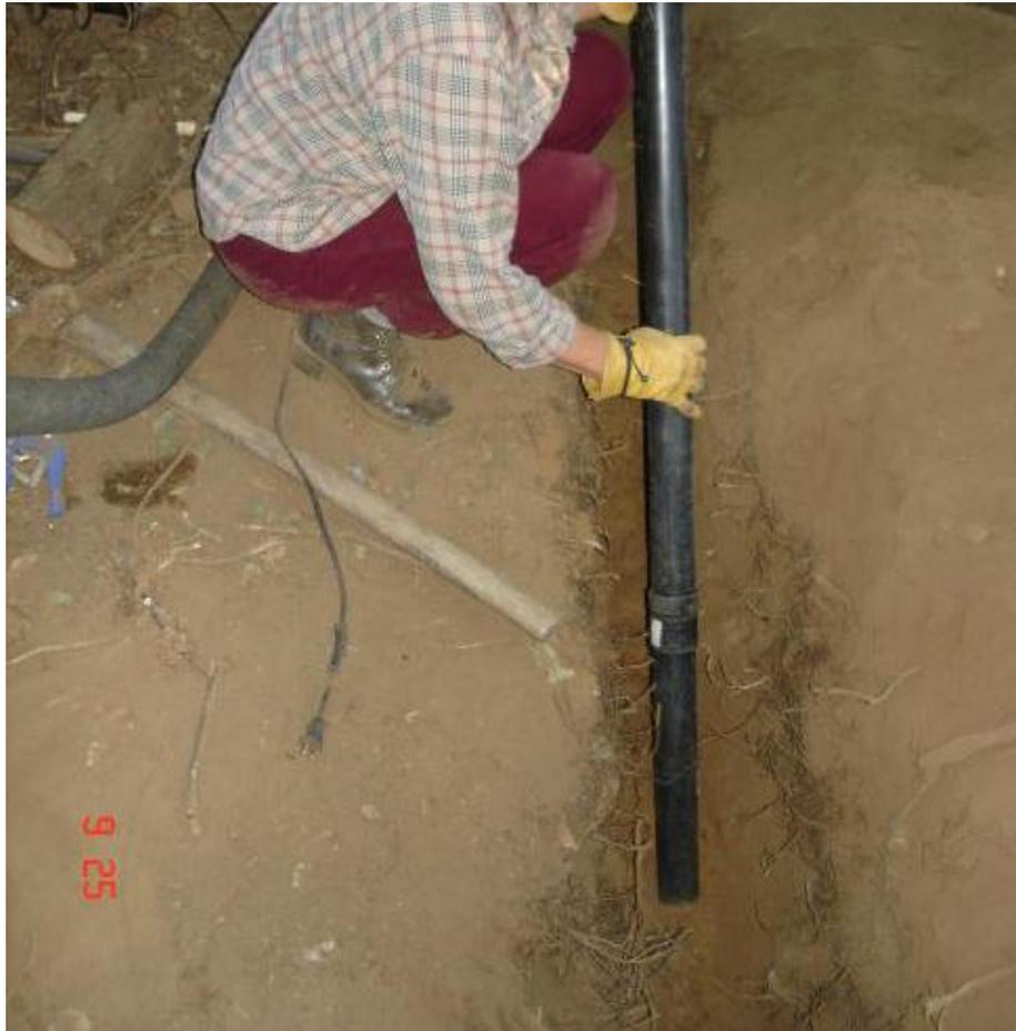
As I stated previously, I thought I'd need to use barbed connectors in the trenches, but later realized that I could pull the pipe up tight, weld the connection, working just inside the trench and then push the pipe in and cover it while holding it down with anything heavy (like large stones or my foot).
