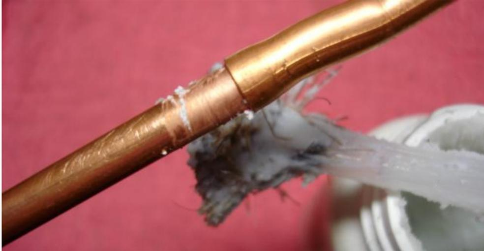
Here I'm applying silver-brazing flux to the tube that will slip inside.
