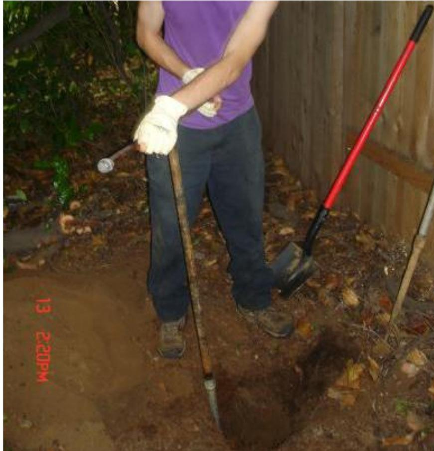
...soon we were down to the end of the extension. We also determined that a bit of water helped the mostly sand adhere better, and made it stay on the auger head while we lifted it to the surface"
